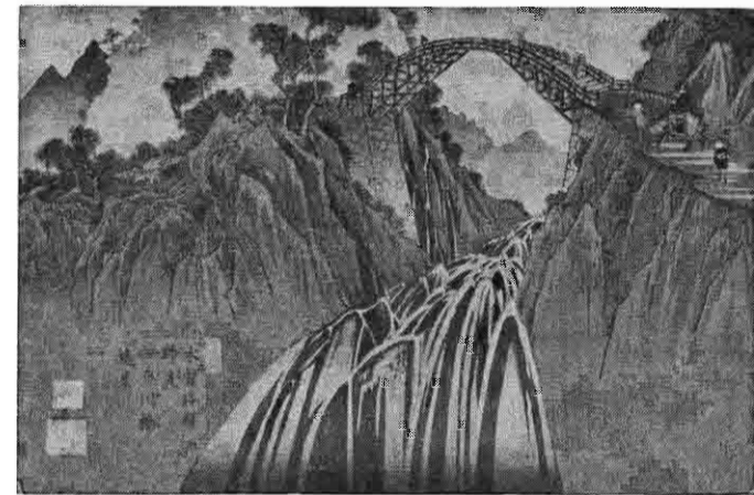
Inagawa Bridge from Views Along The Highway by Yeisen. Underside of the bridge follows the contour of Mt. Fuji. (Floating World)
