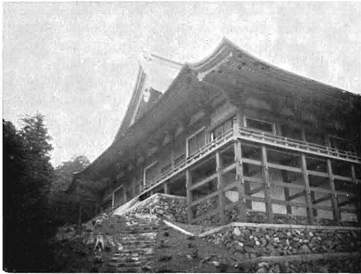
The Yokawa-Chudo, originally established by Abbot Ennin and recently reconstructed.
