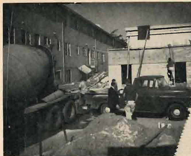
VIEW OF CONSTRUCTION
